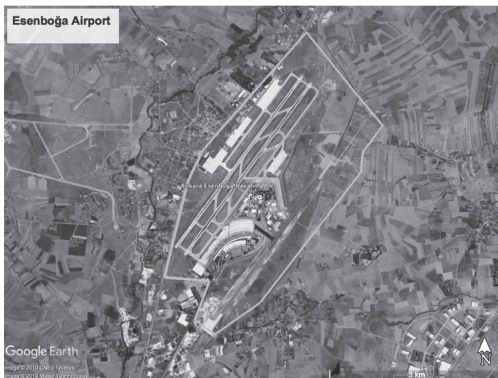
Figure 1. General view of Esenboğa Airport
