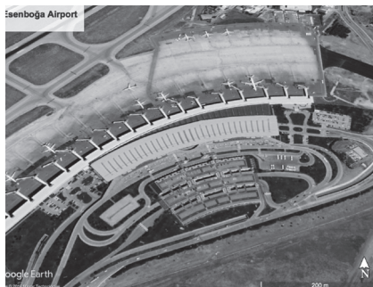
Figure 5. Esenboğa Airport Terminal Rooftop Area
